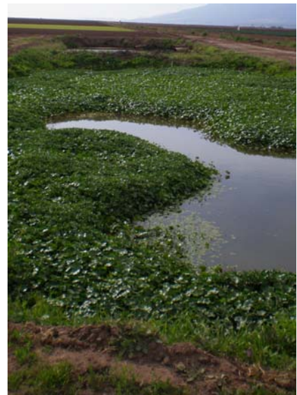
Figure 3. Example of a Vegetated Treatment System – dual ponds and floating pennywort.
